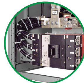
Fig. 13: Ground and neutral disconnect links
