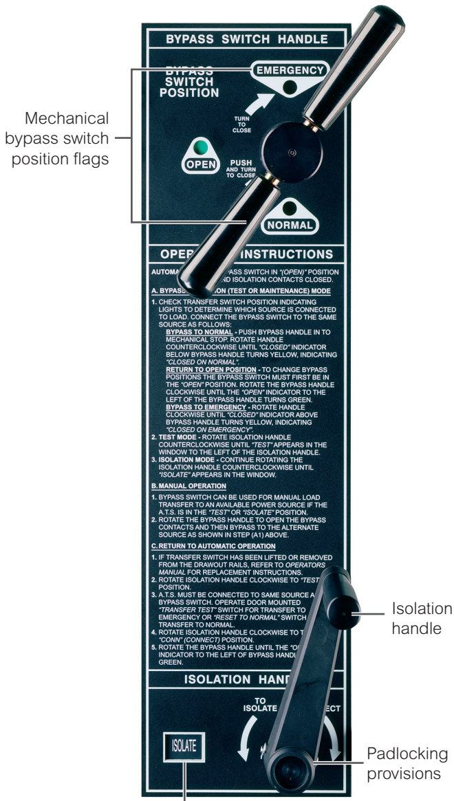
Mechanical isolation handle position window (connected/test/isolate)
